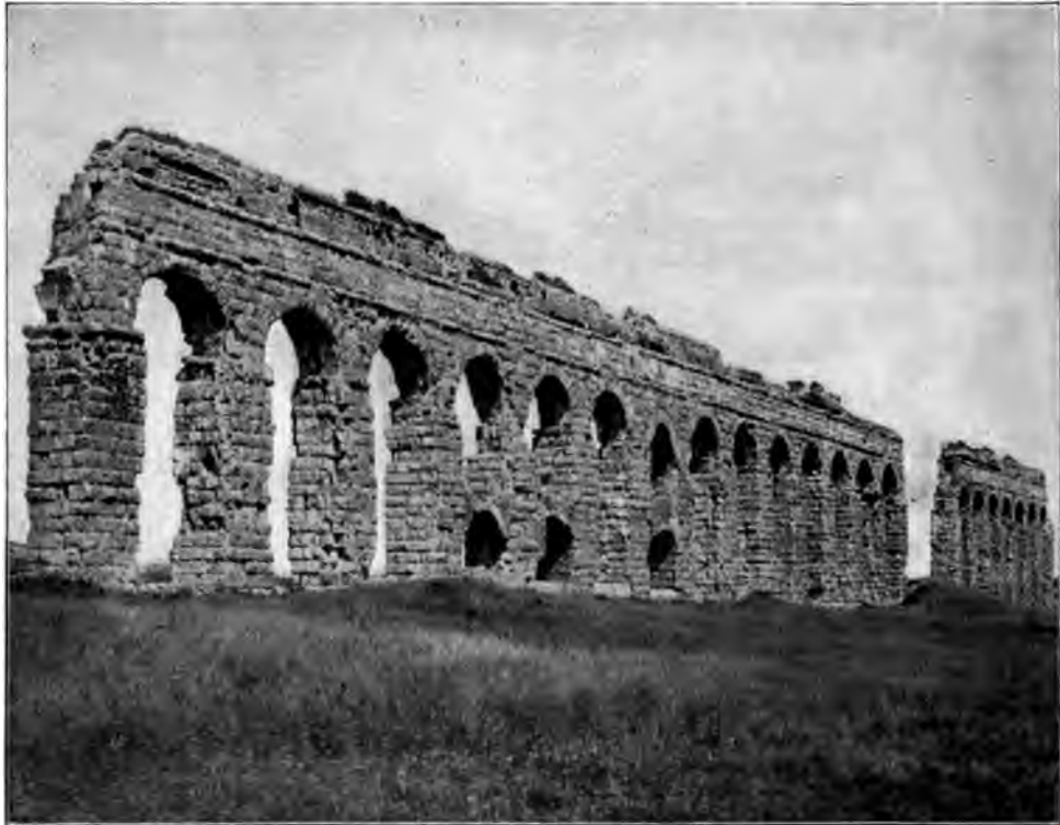
CLAUDIA, OF DIMENSION STONE, AND ANIO NOVUS, OF BRICK AND CONCRETE, ON TOP OF IT. 1
